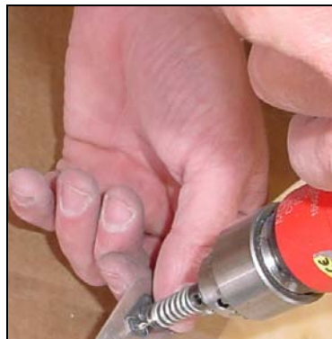
Screw nutplate on back side
