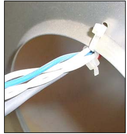
Alternative to using grommets; double tie wrap technique.
