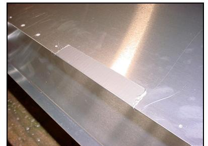
Use pieces of duct tape to hold the skin flush with the edge of the flange (channel)
