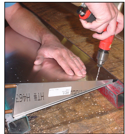
Start at the back and work towards the front.
