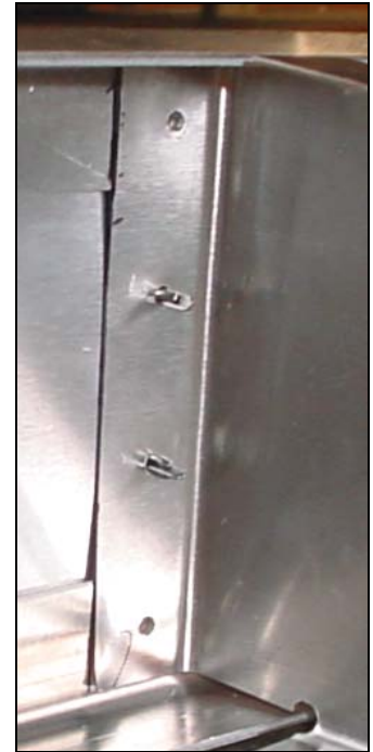
View of rib flange.
