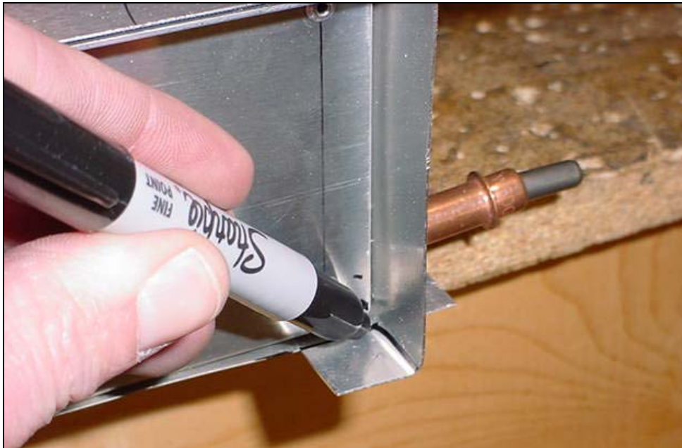
Trace the spar on the flange.
