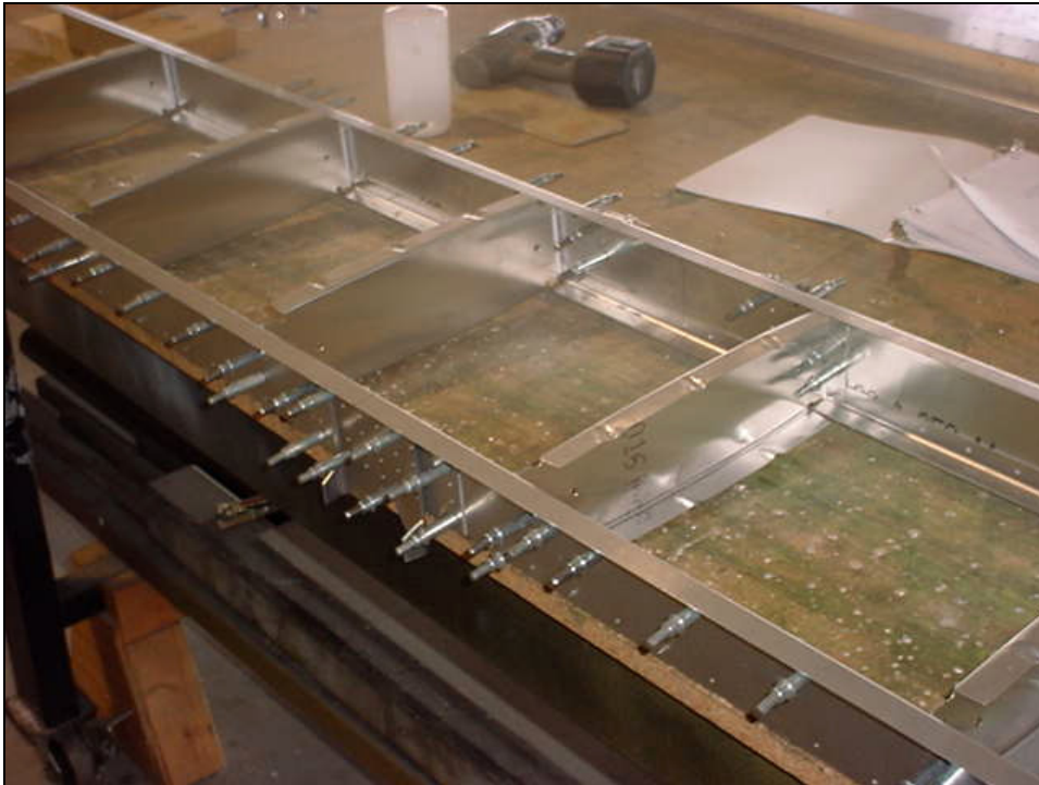
Drill & Cleco ribs to spar.
