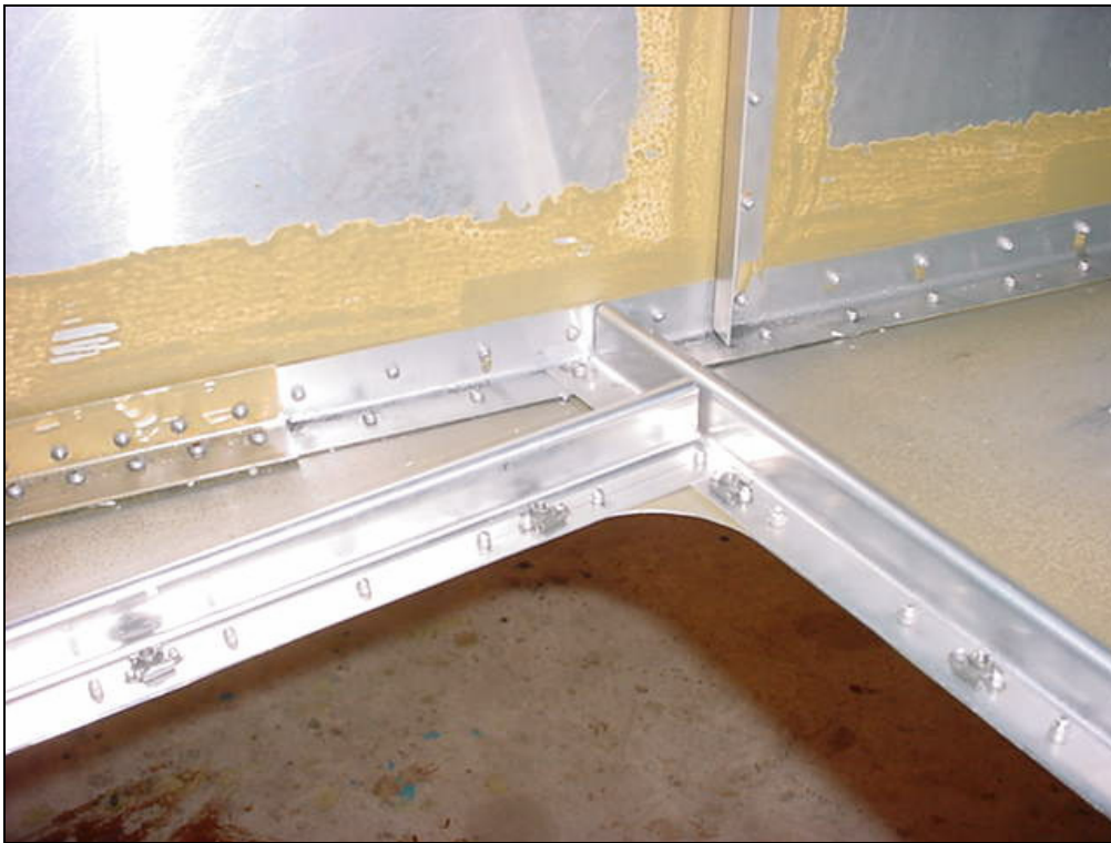
First locate the position of the nut-plates, then layout the rivet pitch (side Z angles).
