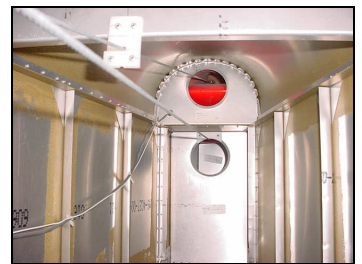
Access to lower cable fairlead on 6B1-1
