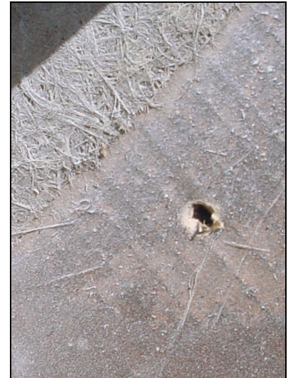
1/4" hole in bulkhead.
