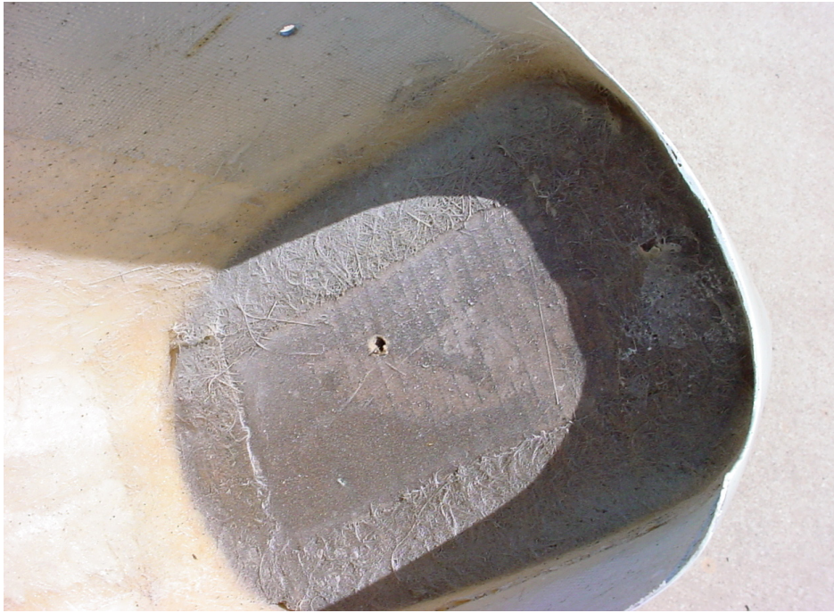
1/4" hole in bulkhead.
