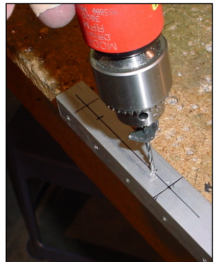
Layout the bolt holes. Pre-drill.
