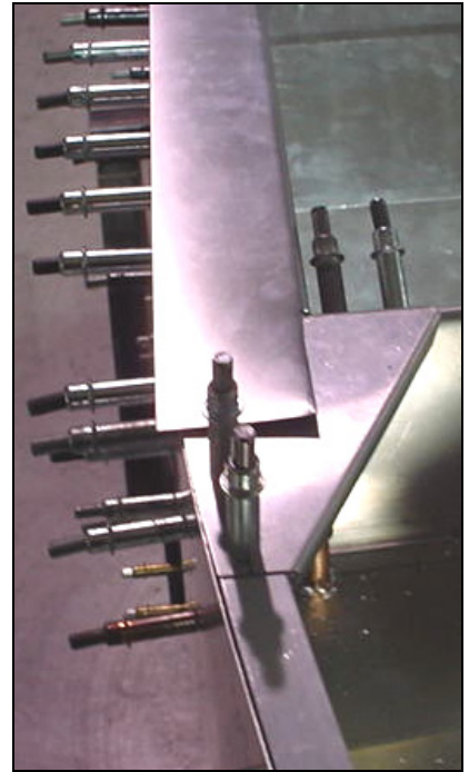
Aft overlap on top of gusset 6B15-1
