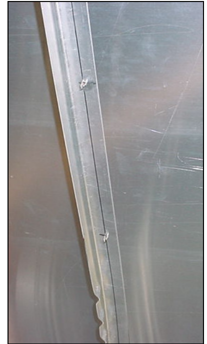
First layout out the location of the horizontal L angles down the vertical L angle, Pre-drill the intersection holes with pilot holes.
