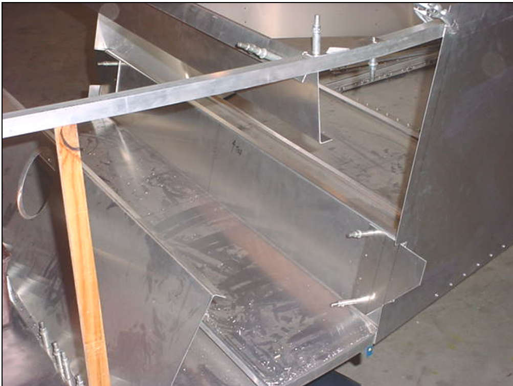
Rear fuselage with rear frame channel 6B5-2 installed. Photo looking towards the rear.
