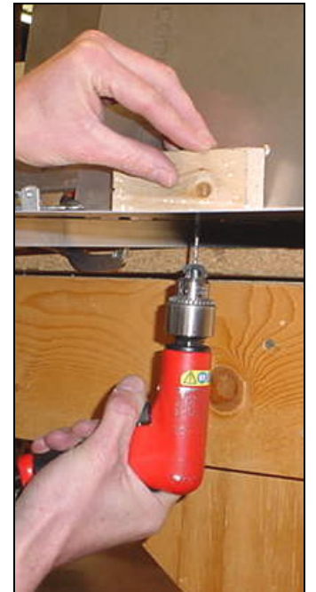
Wood backing block on top side.
