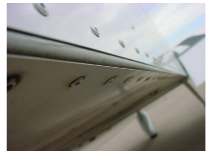
At the HT frames the bend radius of the Longeron is visible.
