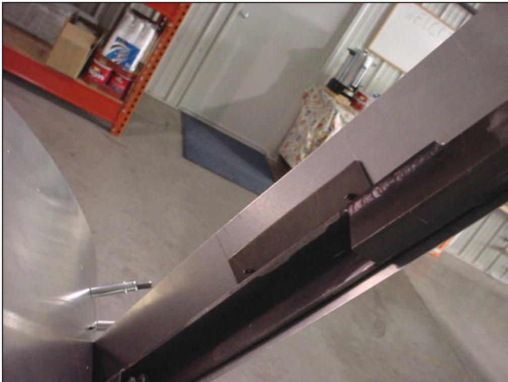
Inside view of clecoes on welded tab.
